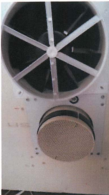
Bild 4: Ventilator removed, heatexchanger pulled out
